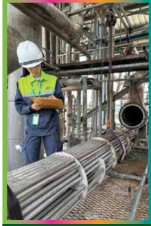
A Yayasan KLK scholar inspecting the condition of vessels (shell and tube heat exchanger) during her internship programme
